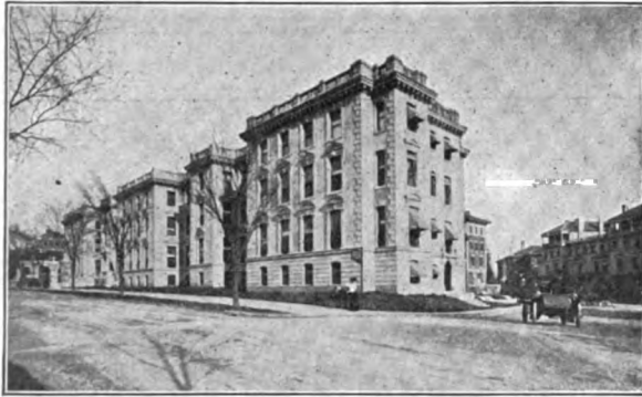
Hotel from N. W. corner, showing Regent Circle entrance to Auto Garage.
